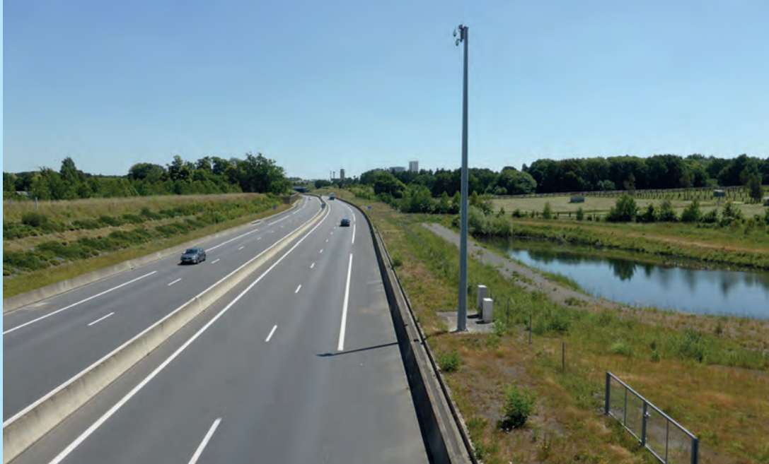
Îlot de gestion. © Cerema
