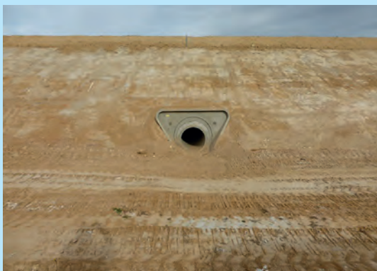
Terrassement routier. © Cerema
