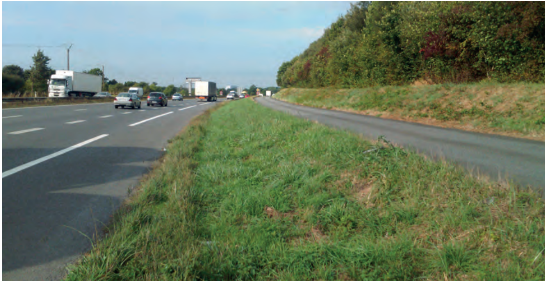
Terre-plein central. © Cerema
